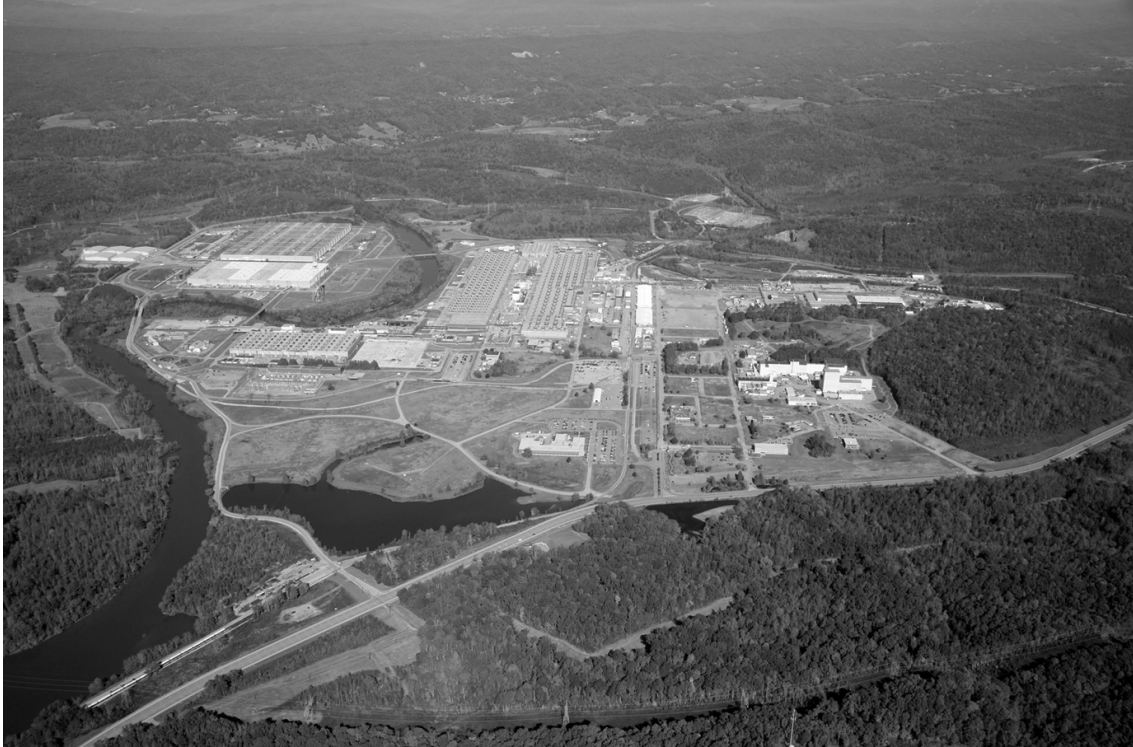
Fig. 3.1. East Tennessee Technology Park.
