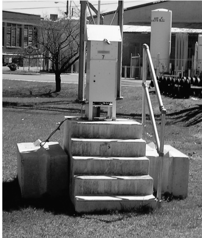
Fig. 3.15. ETP ambient air monitoring station.
