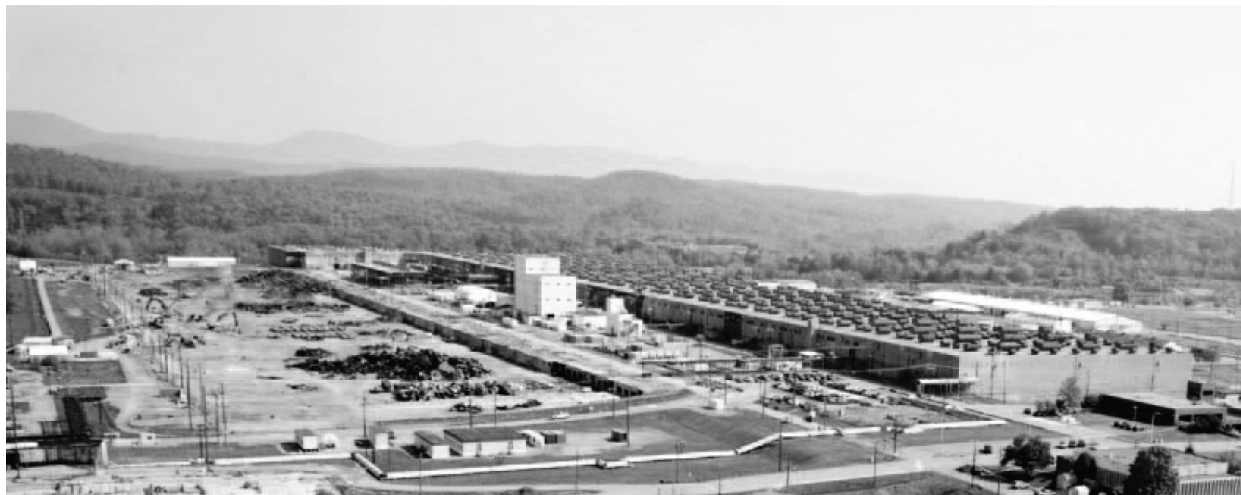
Fig. 3.66. The K-25 Building after demolition of the west wing.
