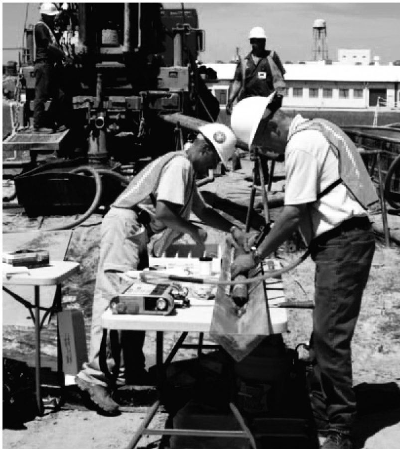
Fig. 3.67. Drilling exploratory boreholes near the K-1401 area.
